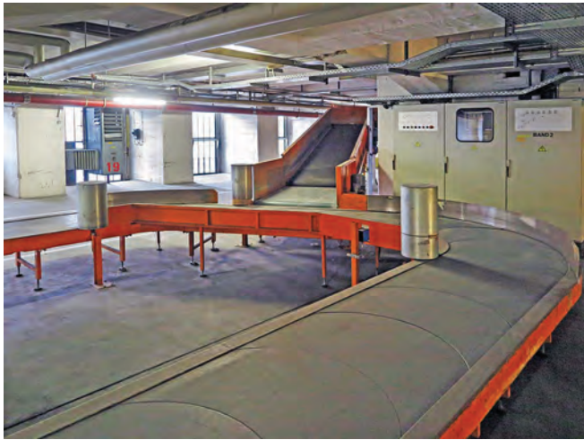
Baggage belt beneath the huge cantilevered roof of the departure area. Photo Clive Penfold
